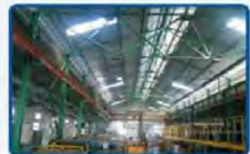
Plant Inside View
