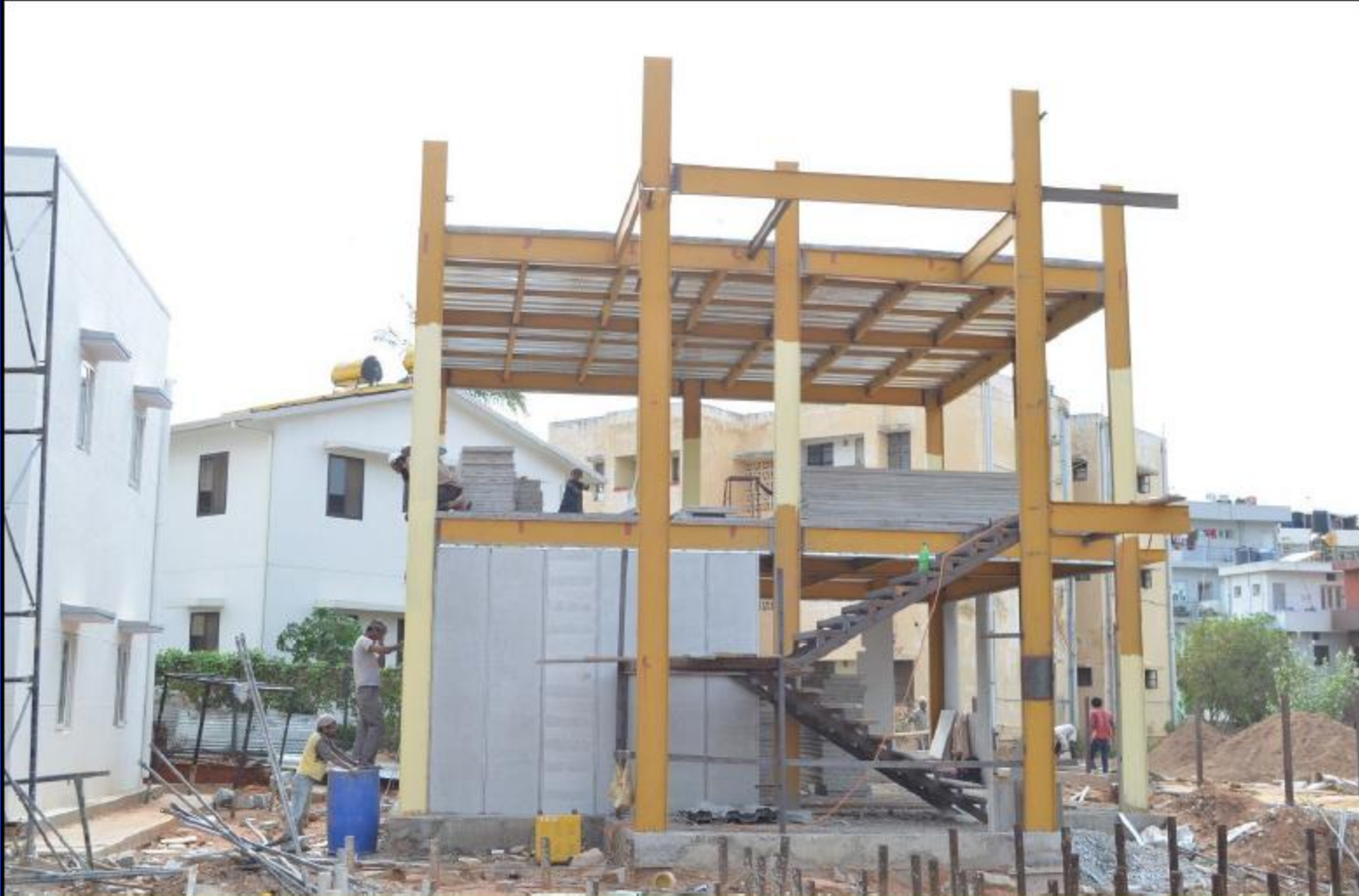
Steel skeleton with Aerocon panel infills
