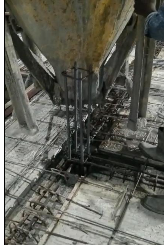
Beam – column - slab wet jointing
