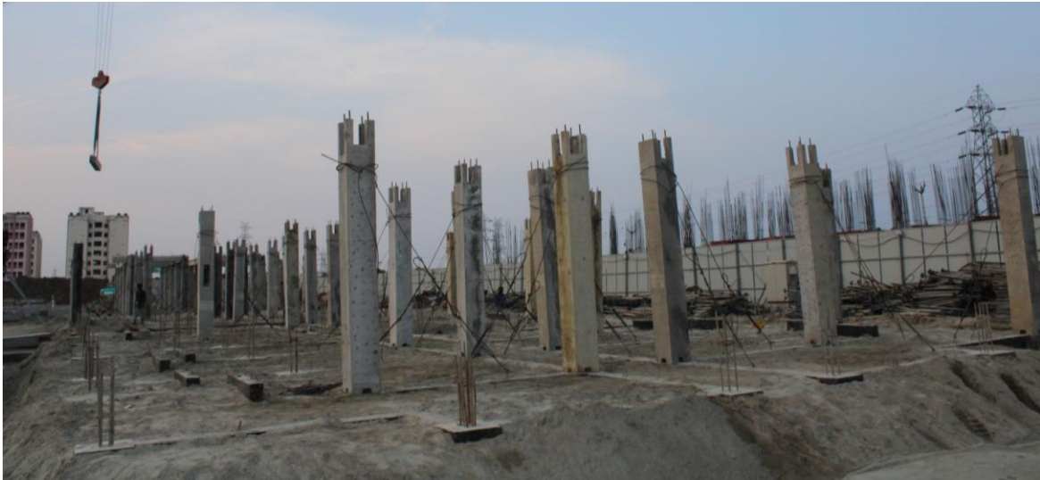
Erected Precast columns with notches and dowels over plinth beam
