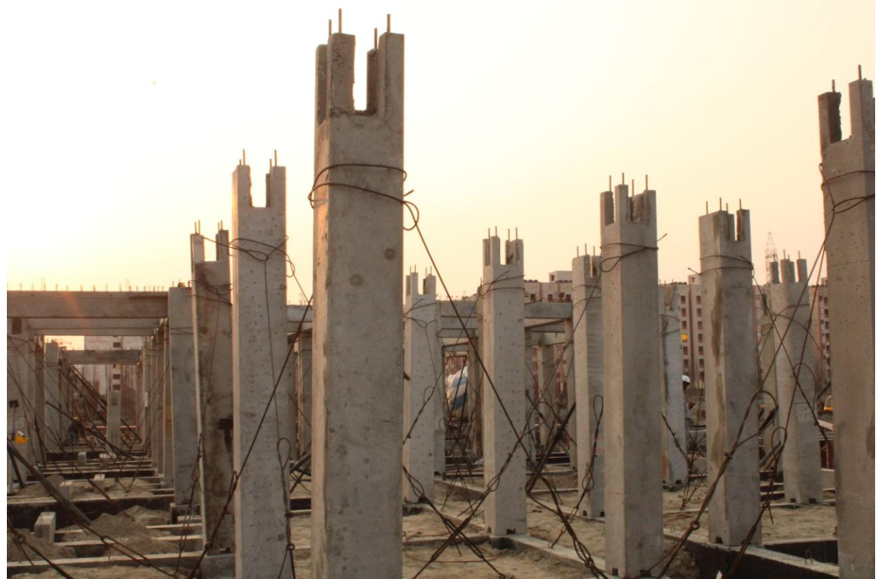
Erected Precast columns with notches and dowels over plinth beam
