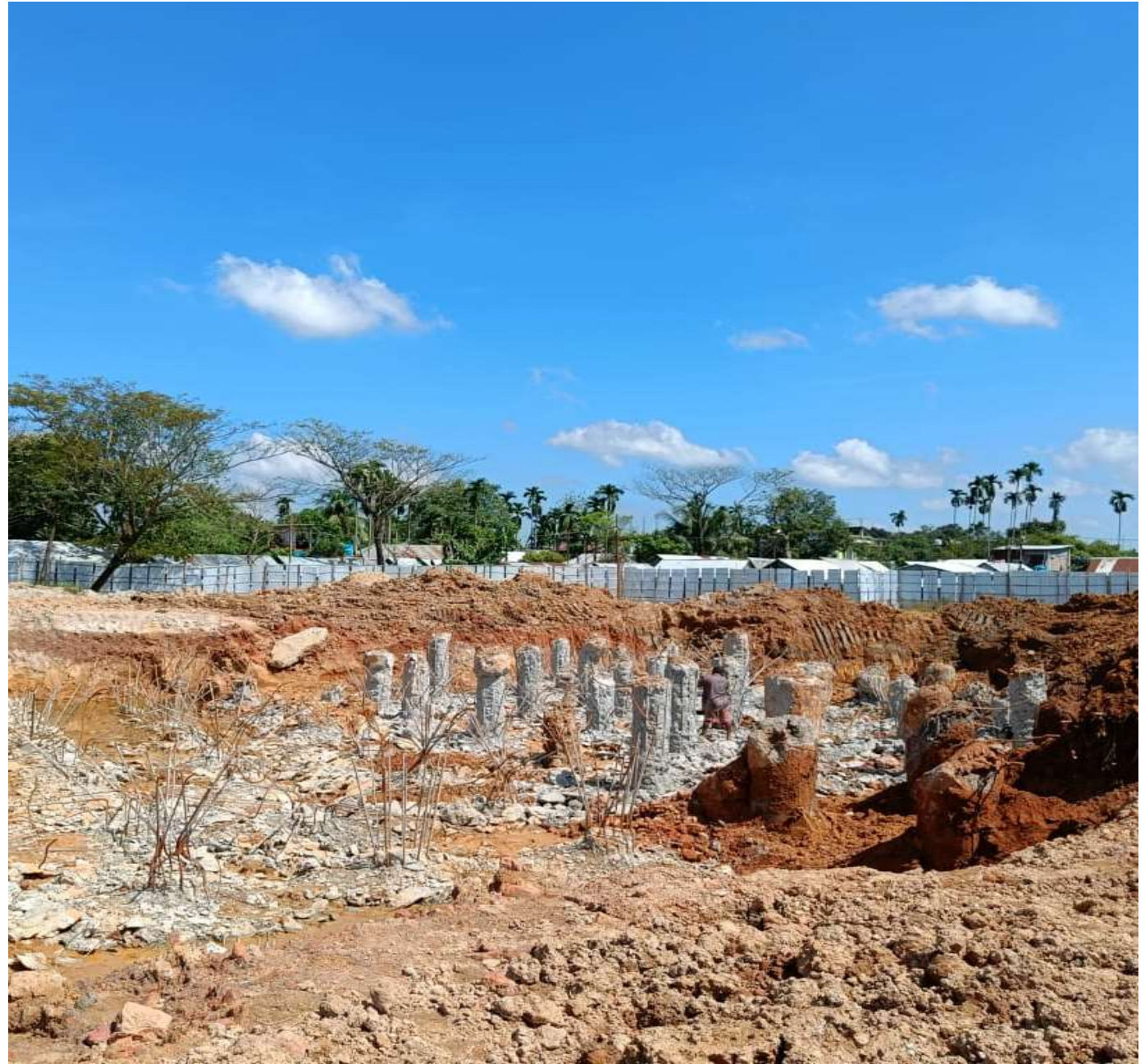
Excavation and pile head breaking
