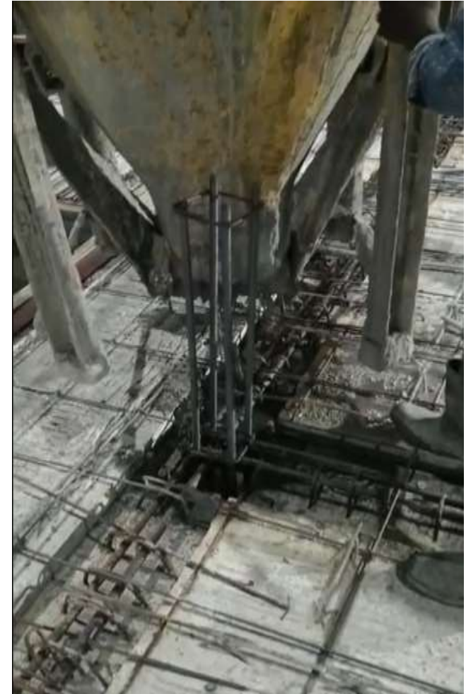
Beam – column - slab wet jointing
