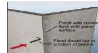
Typical L & T joints with panels
