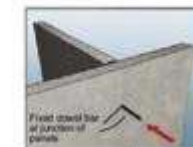
Lock the Panels with each other with the help of steel bar from head
