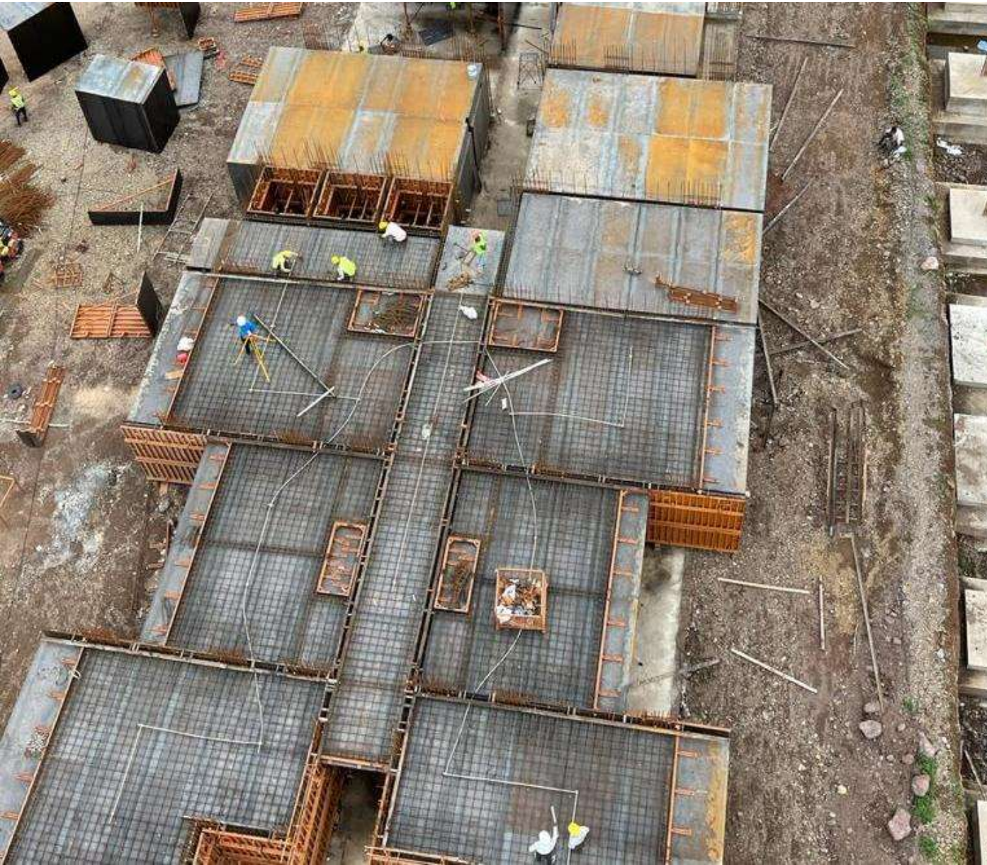
Typical Reinforcement at Slab level
