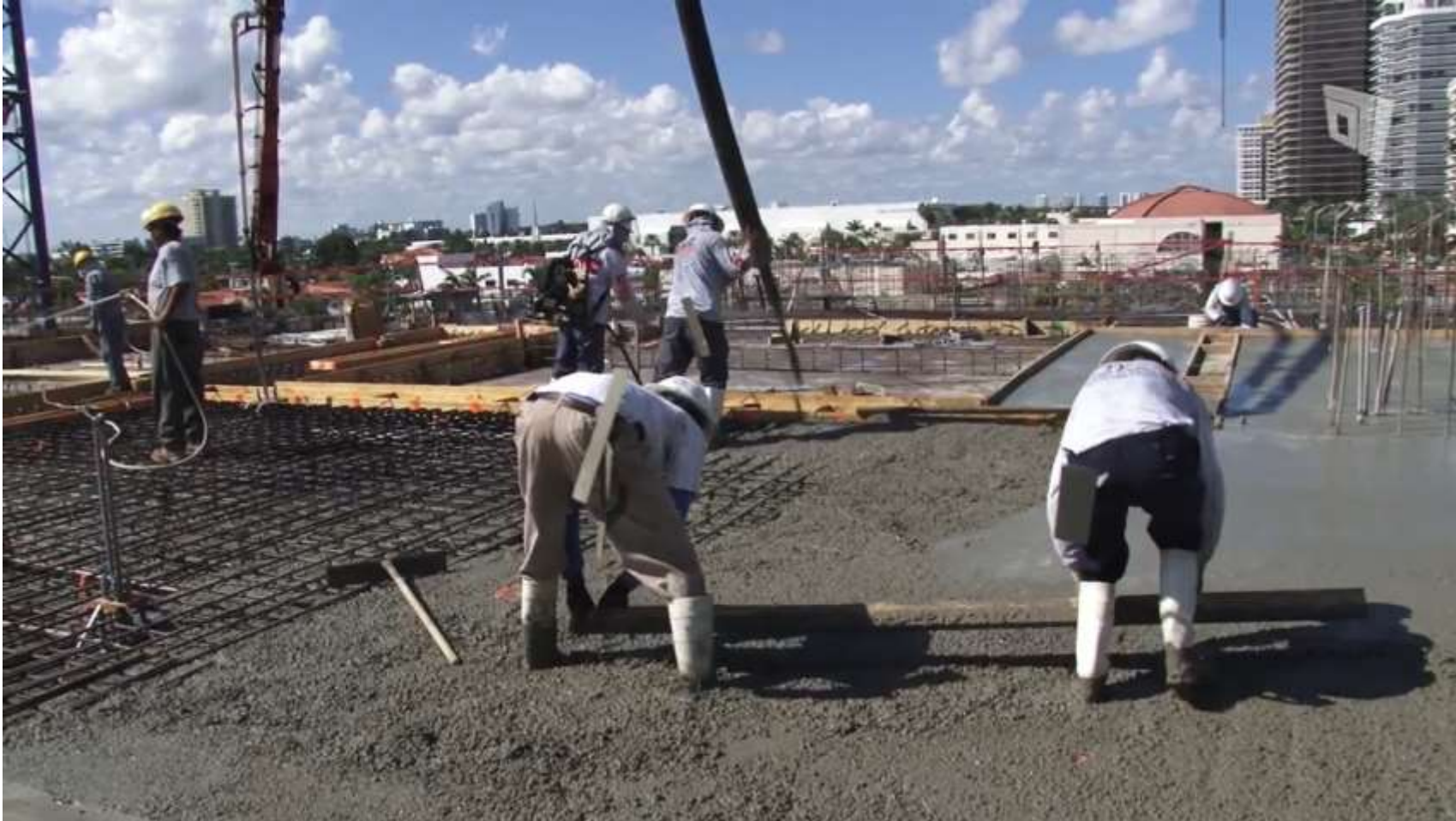
Placement and leveling of concrete
