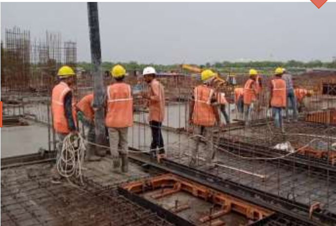
Concreting after Placing formwork
