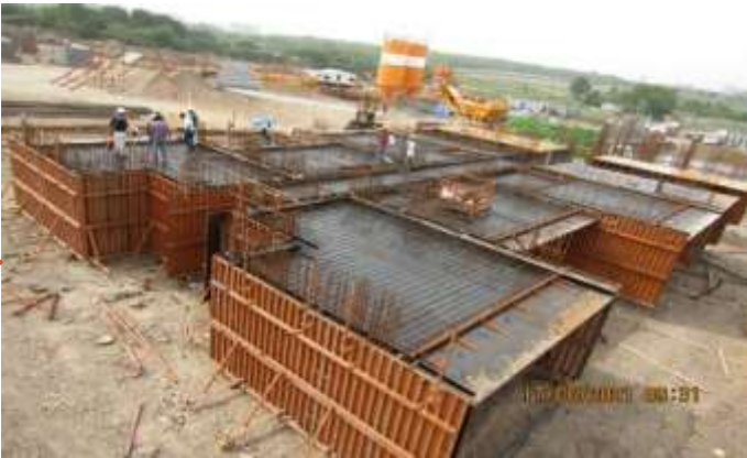
Assembly of Formwork
